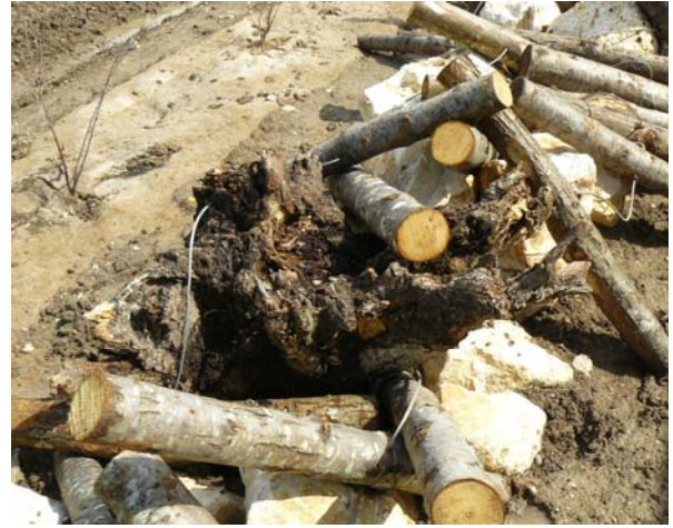
Photo 3: detail of the windrow (rocks and logs linked to one another – A10 DTer SO)
